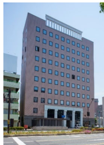
Nagano Central Building
