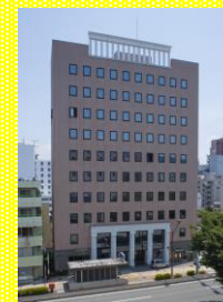
Nagano Central Building
