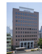
Nagano Central Building
