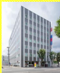
EME Koriyama Building
