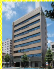
Utsunomiya Central Building
