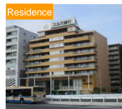
MARE Isogo Building
