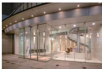
NT Building (entrance)
